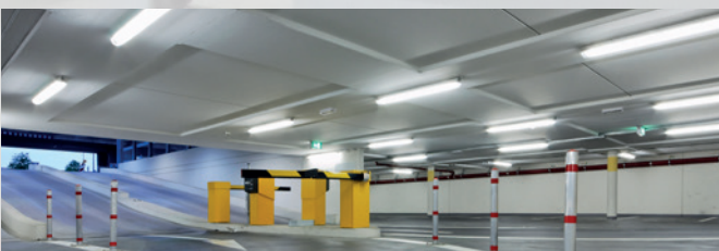
Parkhaus Parking Garage
